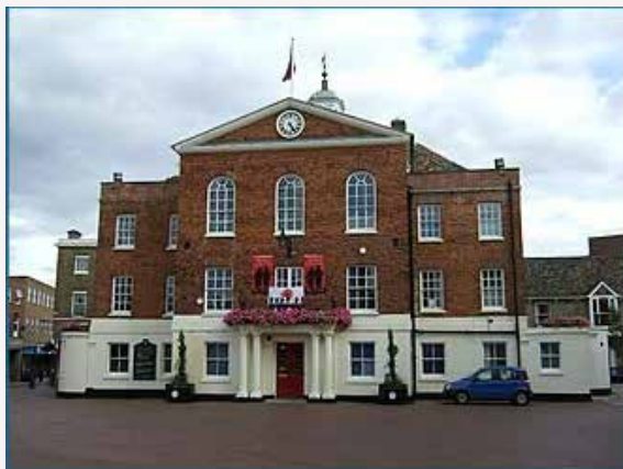
Huntingdon Town Hall, formerly the Court House
